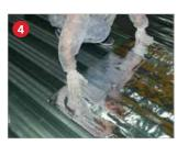
Proceed by rolling the membrane on the decking and simultaneously pulling off the siliconized film.
