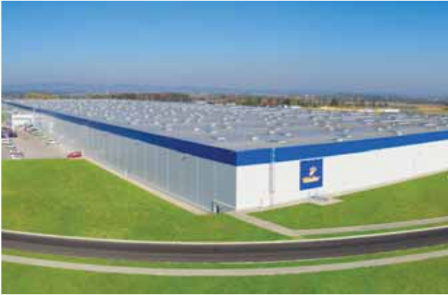
Distribution centre Accolade, Cheb, Czech Republic LOGICROOF V-RP 1.5 mm | 65.000 m 2
