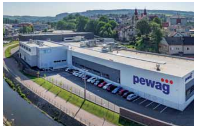
Production hall, Vamberk, Czech Republic LOGICROOF V-RP 1.5 mm | 9.800 m 2
