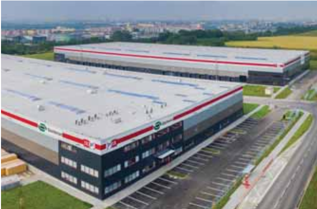
P3 Park, Hall IX and X, Horní Počernice, Czech Republic LOGICROOF V-RP 1.5 mm | 25.000 m 2
