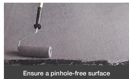
Wetting through the fibreglass CSM
